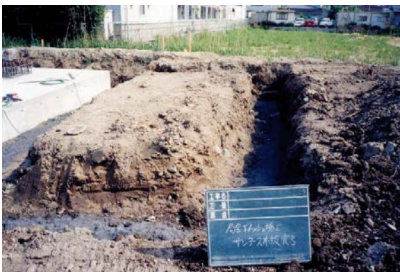
Laying SAN-EARTH M5C *One 25kg bag of M5C will cover approx. 3 meters (width 50cm) .
